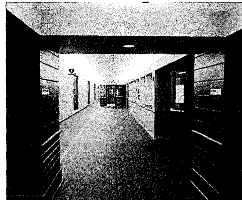
Existing entry corridor for NDVS/SB renovated in 1996.
