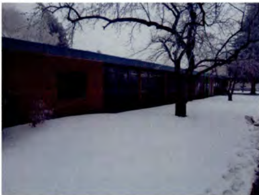
Stanford Centre West Wing showing existing, original window wall system recommended for replacement.
