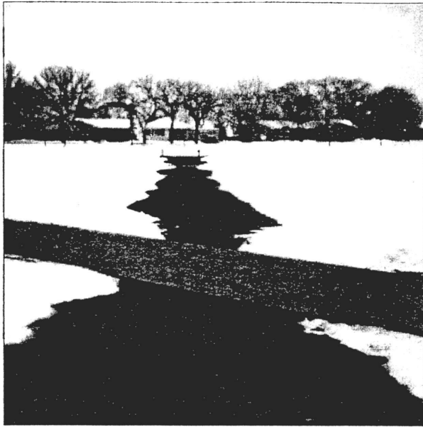
1-30-98 Deteriorated steam lines south side Robertson Hall.
