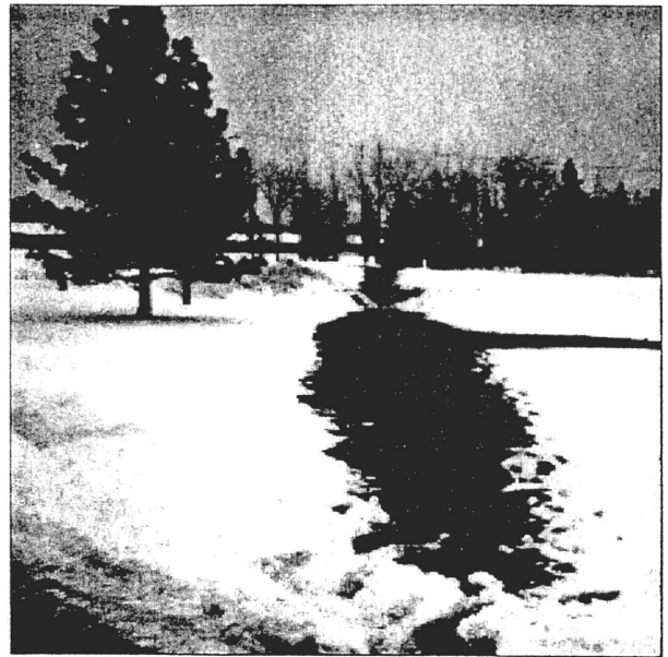
1-30-98 Deteriorated steam lines Blikre Activities Center south to Frank Vertin Field.
