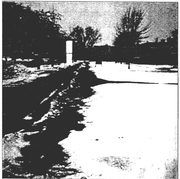
1-30-98 Deteriorated steam lines east of Burch Hall north and south.
