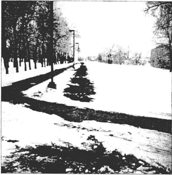
1-30-98 Deteriorated steam lines north of Patterson Maintenance Center to Blikre Activities Center.
